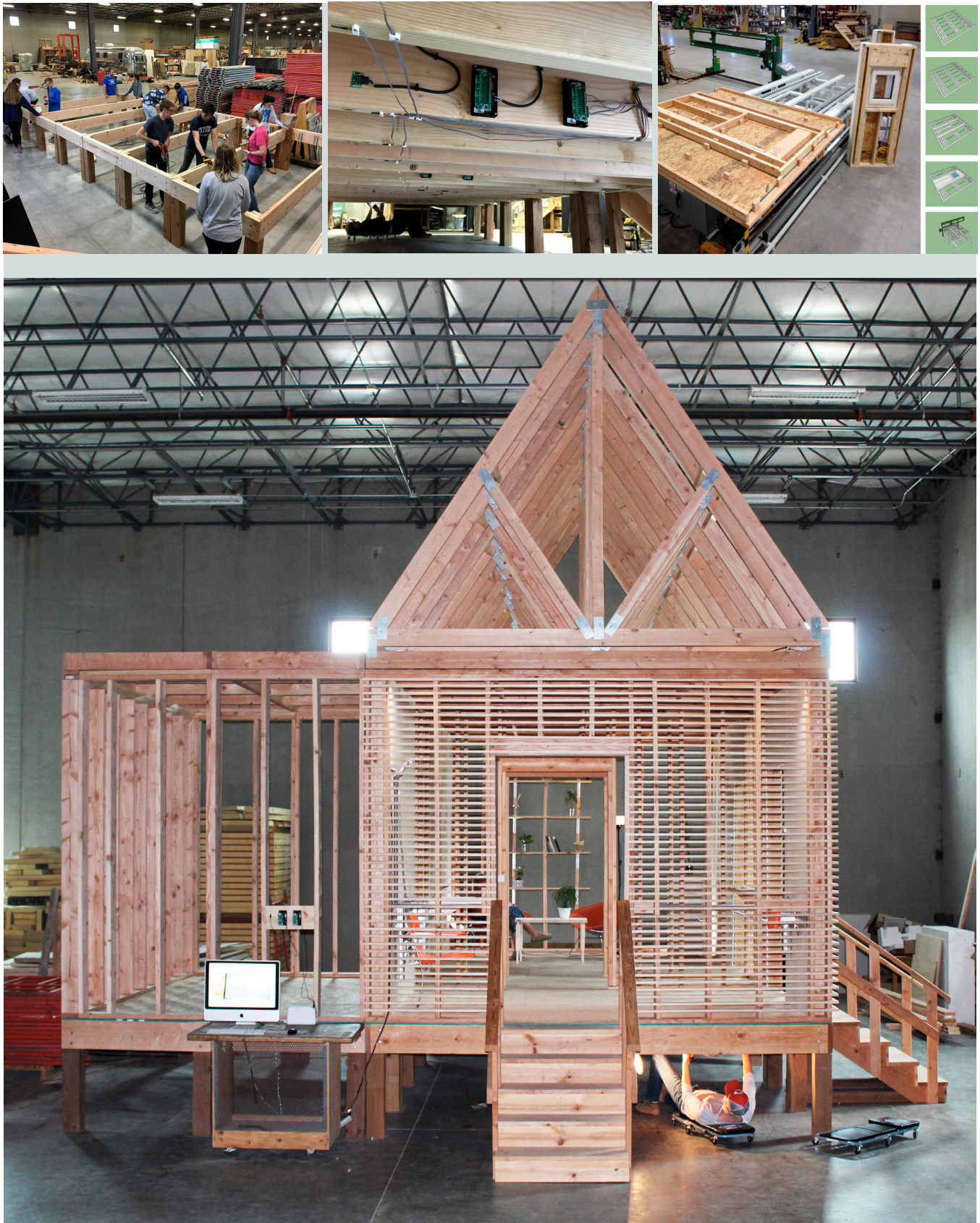
Figure 2. Smart housing prototype constructed in the University of Kansas Design Build Lab.
